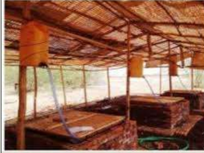
Zero Energy Cooling Chambers (ZECC)
